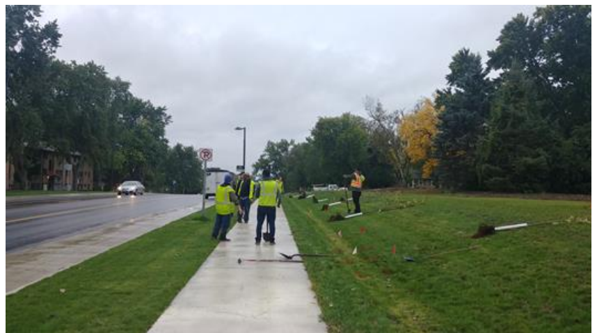
Contractors planting boulevard trees in Hennepin County.
